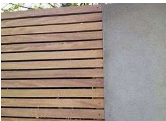
Timber iroko cladding to the pedestrian face of the Armco.
