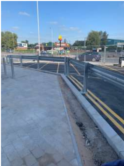
Existing Armco barrier
