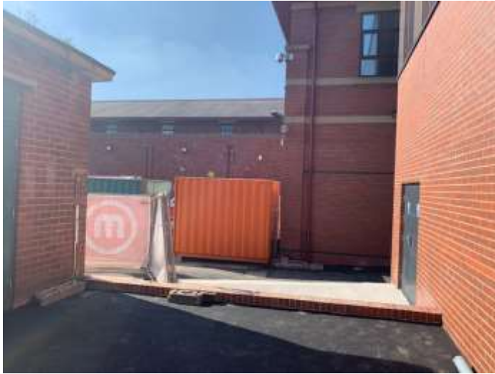
Front elevation of fencing required to block off the view of the service yard.
