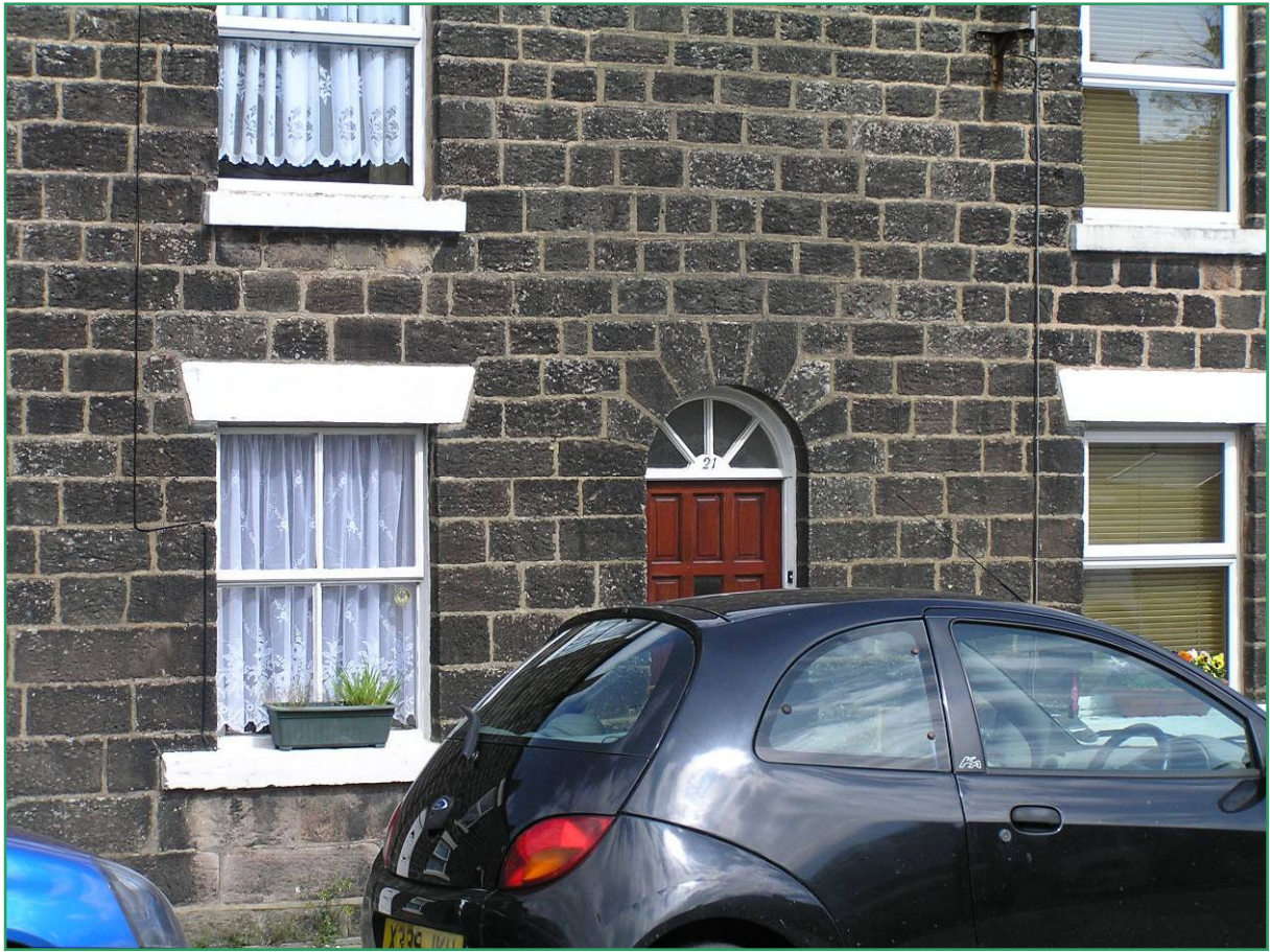
Possibly the only surviving original timber sash window in Abbey Village?
