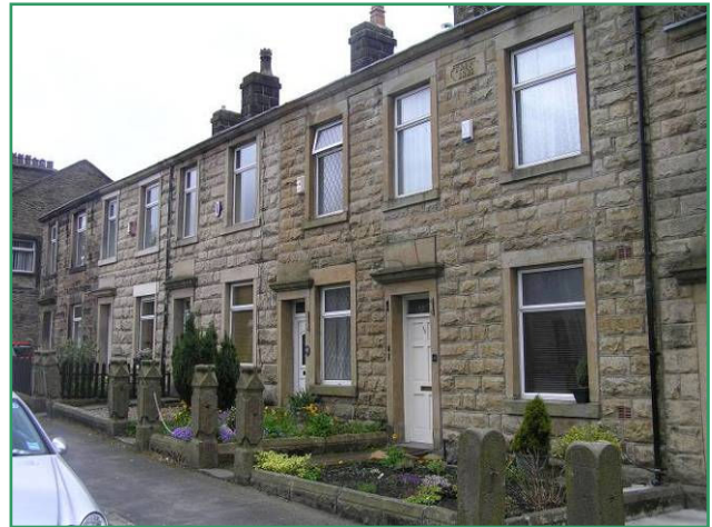
Stone window and door surrounds, front garden walls
